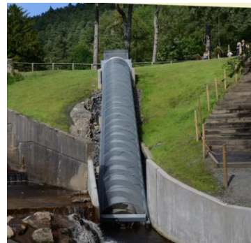
Figure 5-10 Archimedes screw
