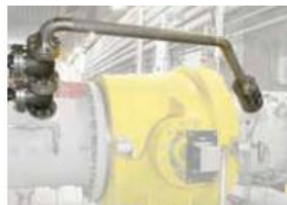
Figure 5-16 Bypass valve
